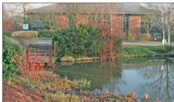
Wetland feature https://www.susdrain.org/case-studies/pdfs/aztec west business park south Gloucestershire final v2.pdf
