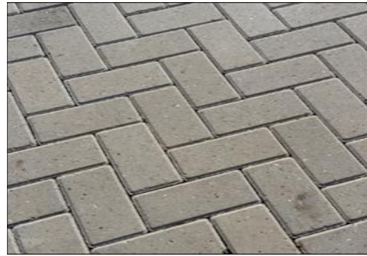
Author's photo of so-called 'permeable paving' which isn't permeable at all; there are no notches in the pavers or gaps between them
