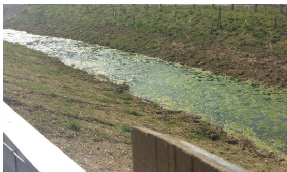
A blockage has resulted in standing water which has developed an algal bloom. The sides of the swales are not correctly planted
